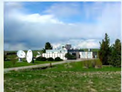
WWV transmitter site in Colorado. The NIST budget request for fiscal 2019 eliminates funding for continued operation of WWV, its Hawaiian counterpart, WWVH, and 60-kHz WWVB. (US Government photo)
